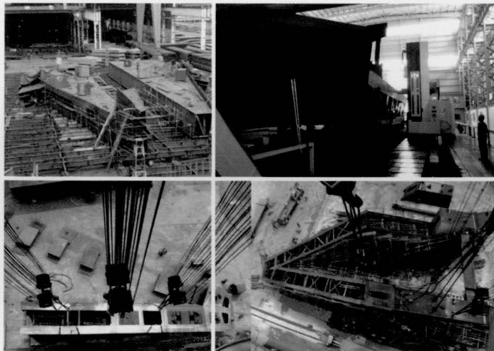
Figure 11: Fabrication, machining and trial assembly of pylon kink.
