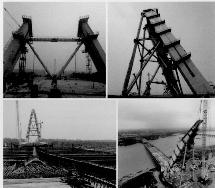
Figure 12: Temporary supports for erection.
