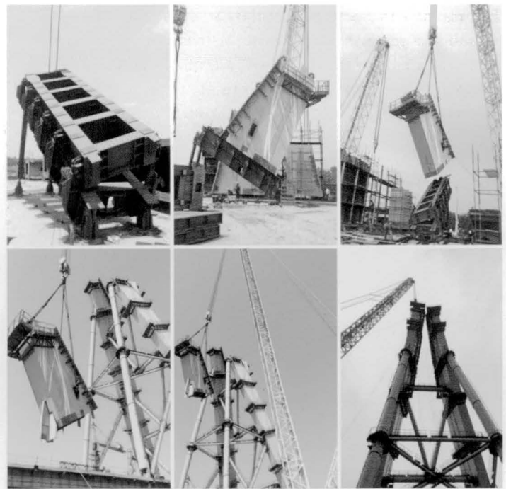
Figure 14: Specially designed turn table for rigging three-dimensionally varying pylon segments.
