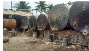
Sodium Silicate factory
