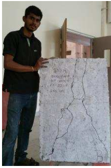
Crack pattern for S3 and S4 slabs
